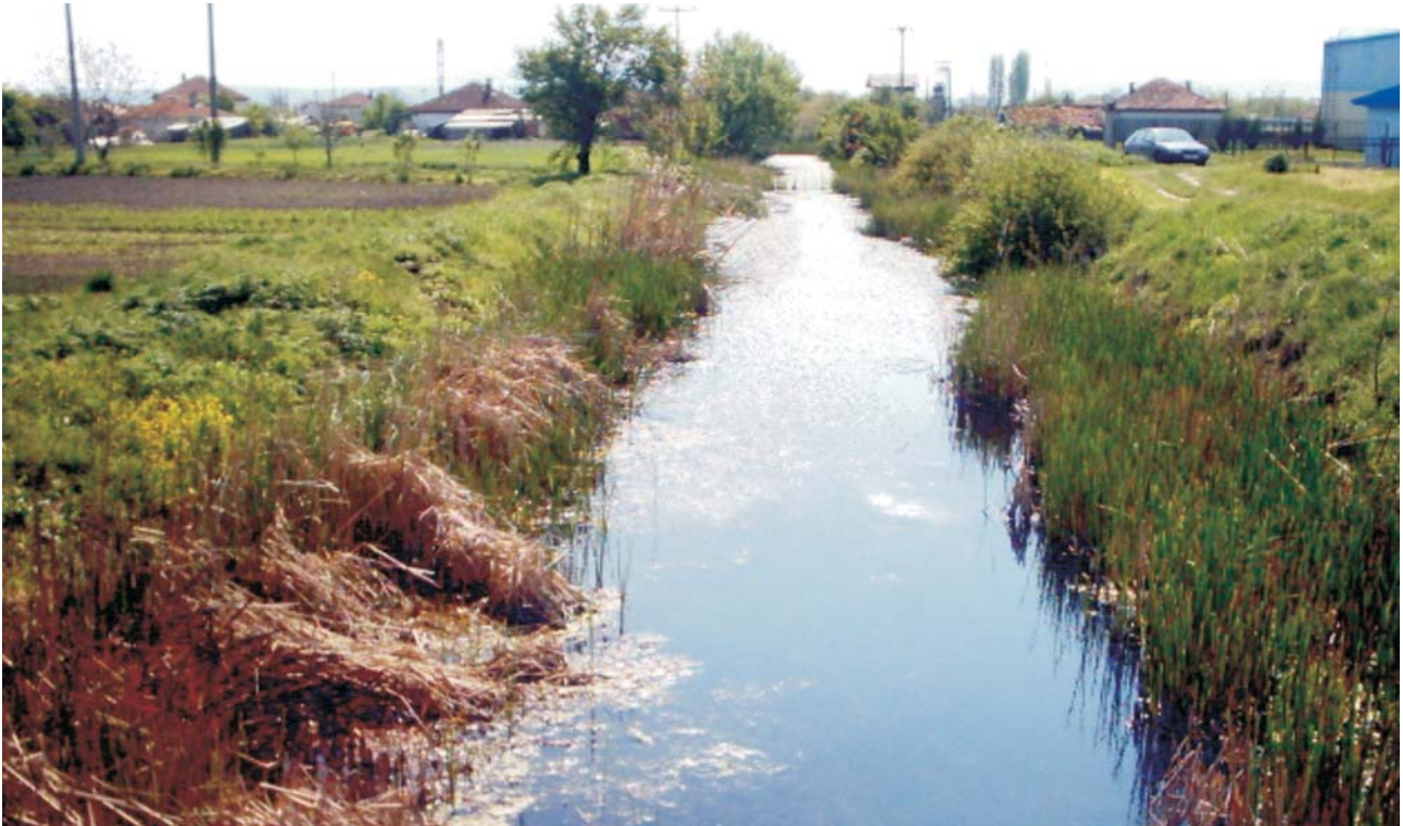
Picture 3. Drainage channel in i.p. Ilinden
